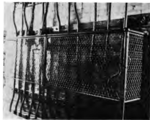
Fig. 6. Guard for Exposed Portions of 6600 Volt Underground Cables.
